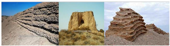
The most essential part of the defensive system was the 23-26 feet high wall. These walls were built using tamped earth between wooden boards, stone and brick mixture, or planks and pilings.
