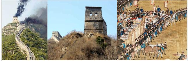
As the name suggests, signal towers were used for military communications by using a beacon in the dark or smoke signals during daytime. Apart from these methods, firing guns, beating clappers or raising banners were also used to communicate. The signal tower were built on hilltops for better visibility. The lower levels of the signal towers were used as rooms for soldiers and storage, and also as sheepfolds and stables.
